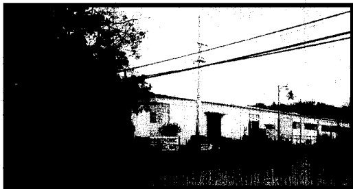
Puerto Rico Facility
